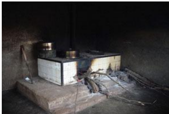
The original Kitchen
