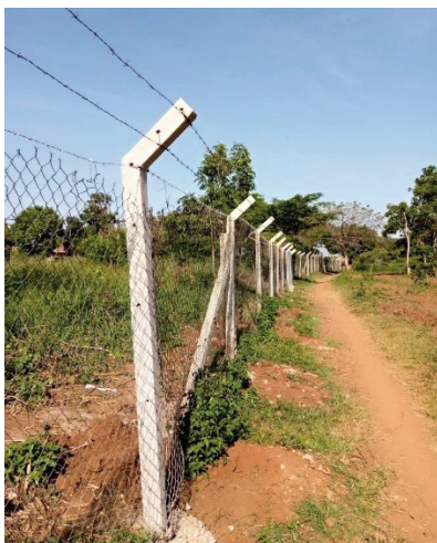
A new fence was constructed at Budaka with concrete posts and metal fencing to stop theft, protect children and to keep out wandering animals like cows.
