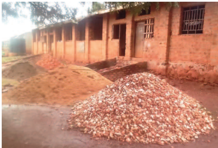
Improved classroom access under construction at Kigulya
